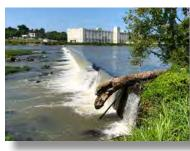
Danville's City Council has recently voted on a **Dam Removal Project** to remove the Long Mill Dam located at White Mill. With the mill having been shuttered for several years, the low-head dam no longer serves its original purpose -- to pond the river water and funnel it through the mill.
