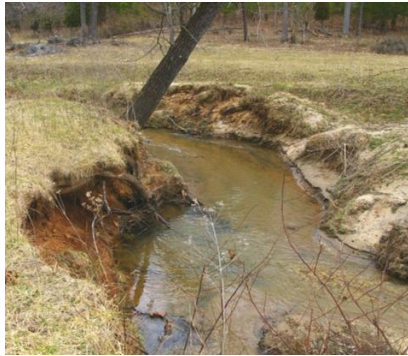
Degraded riparian area
